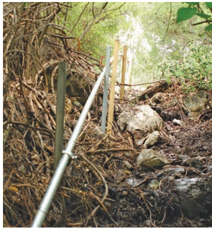
A drive pipe heading downhill with a fall of 35 feet, which creates the force to run the water hammer. No oil or gas needed to pump water uphill. It gets no greener than that.
