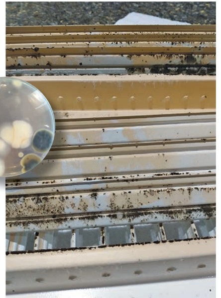
Above: One of the vents before being cleaned with bleach. A petri dish (inset) shows the positive test result (i.e., spores) from the vents in Heninger's bedroom.
