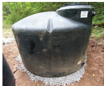
Level and ready for the water.
