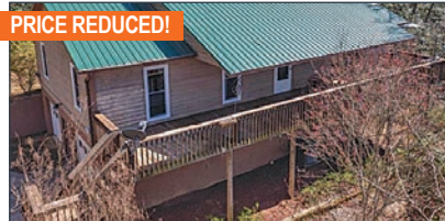
PRICE REDUCED! FAIRVIEW PRIVATE HOME 3BR2BA, 2,359 SF, 1+ AC. Open floor plan on main. Updated BA on main, wood floors, newer fridge. No HOA, no restricts, only $90/qtr rd maint agreement. $457K
