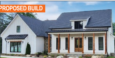
PROPOSED BUILD FAIRVIEW! 38 acres on Old Fort Road. $1.75M Farmhouse style, 3,746 sq ft Call Jenny 828-779-4473
