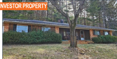
INVESTOR PROPERTY INVESTORS! 3 BR/1BA, 2.5 acres. New roof! Great bones, needs roof, cosmetic fixes. Beautiful property w/ stream & M land. Could split into sev lots. City H2O runs in front. $375K Call Jenny 828-779-4473
