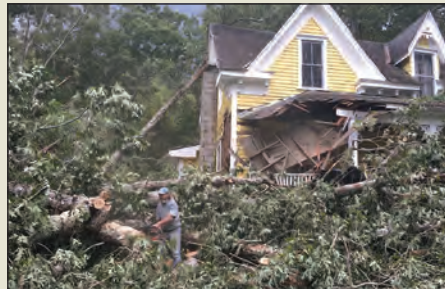
Connie purchased the Ashworth house in 1973 and dubbed it "Mayhem Manor." In September of 2017, Hurricane Irma wreaked some mayhem of her own when a massive old tree crashed down on it. (above) Despite the odds Connie was fine, and her son Mike, a builder with a love for the old, rebuilt it to stand in even more glory than its past. (below) The house is listed in the book Cabins and Castles, The History & Architecture of Buncombe County, North Carolina , originally published in 1981.
