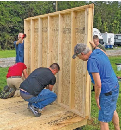
South Carolina volunteers from Sheds of Hope building a shed for The Village
